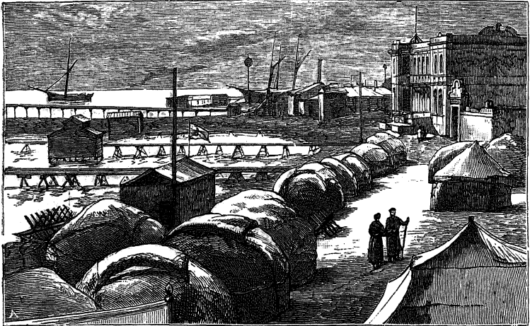
GOVERNOR'S HOUSE AND STORES AT KRASNOVODSK.
